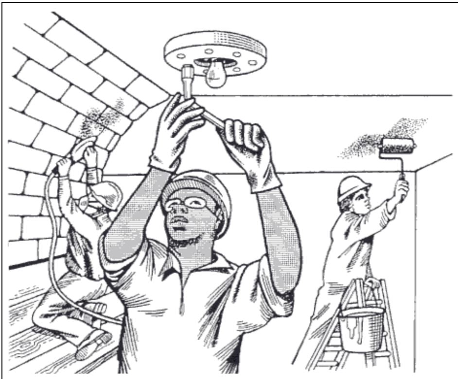
Figure 39. Where possible, workers should not work on surfaces above their heads, as this increases the strain on arms, back and neck
