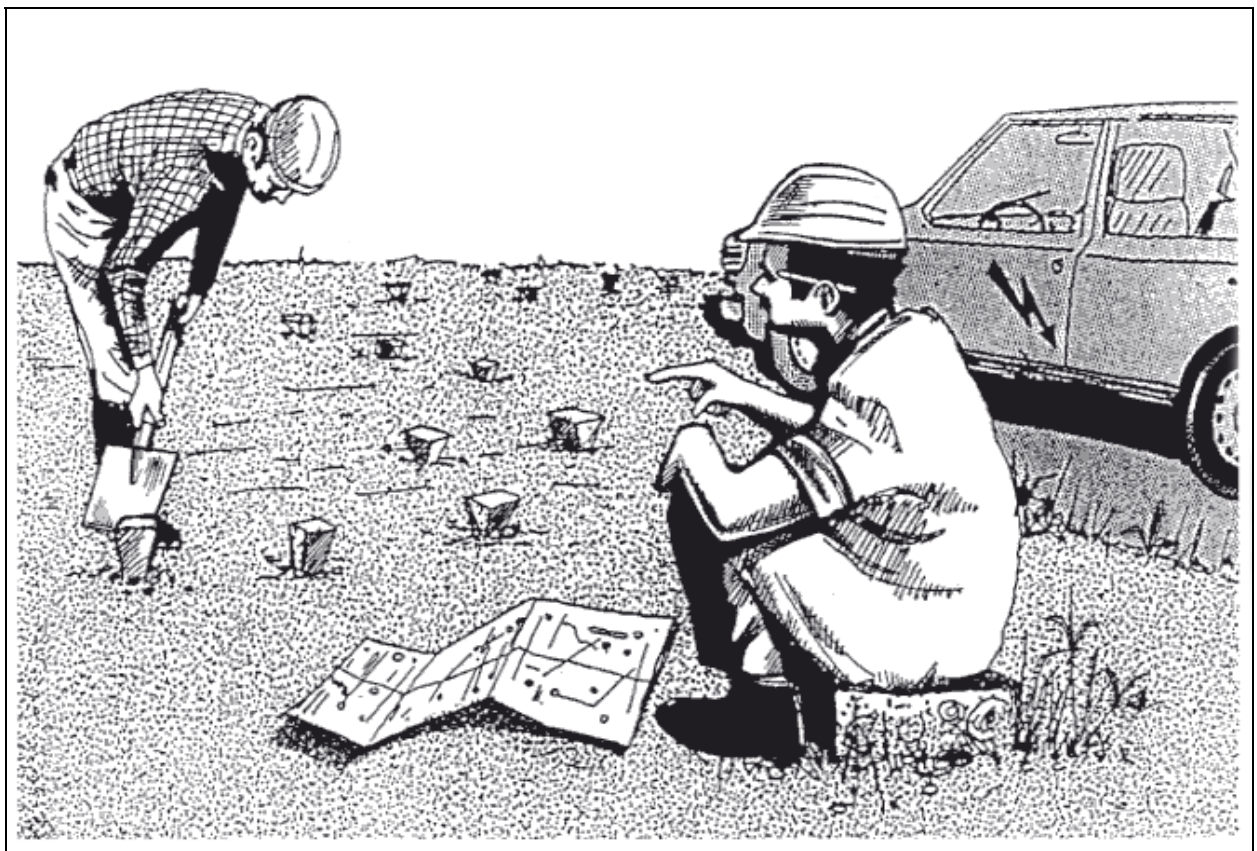
Figure 12. Locating buried electrical cables from a plan and marking their position
